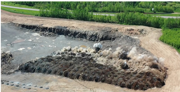
Figure 4. Controlled rock movement during blast.
