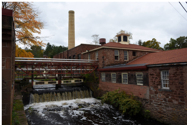
Figure 2. The Simsbury, Connecticut, manufacturing facility supports global R&D.
