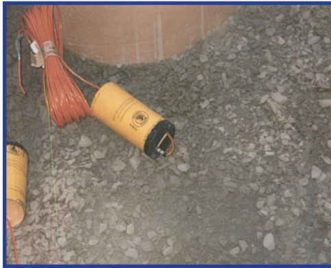
Figure 132 - Primer assemblies awaiting loading.
