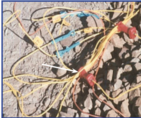
Figure 139 - Tube partially out of connector block.
