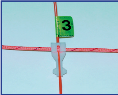
Figure 66 - Proper J-Hook connection.
