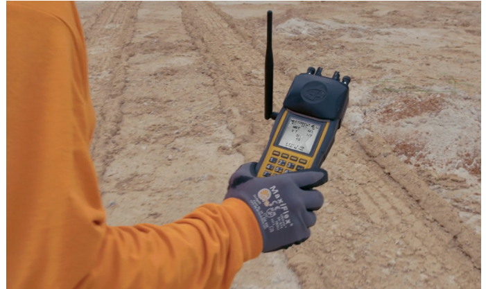
Confirming the accuracy of the hole position.
